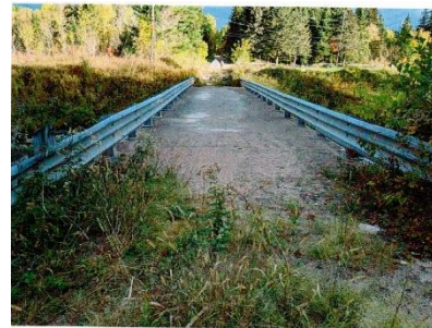
South Approach Looking North
