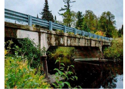
South Pier - Looking SE
