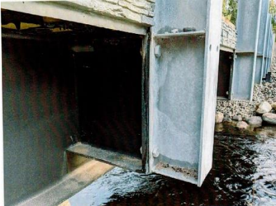
Post to Beam Connection
