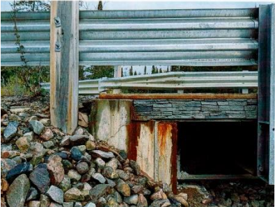
South Abutment Wall, East Elv
