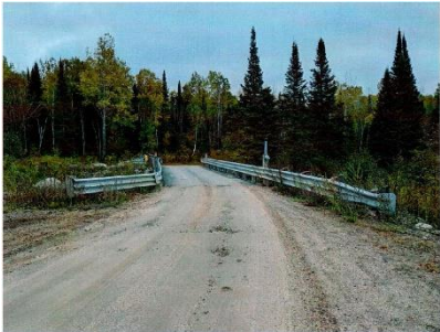
South Approach Looking North
