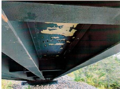
Soffit of East Space
