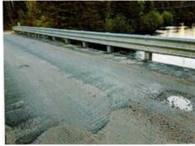
Deck Looking Northeast
