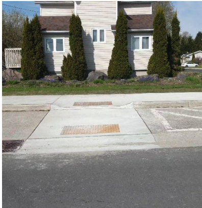
New curb ramps and sidewalks installed for the Lion's Head Sidewalk Project
