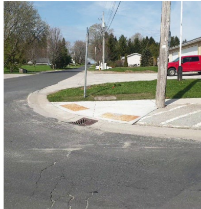
New curb ramps and sidewalks installed for the Lion's Head Sidewalk Project
