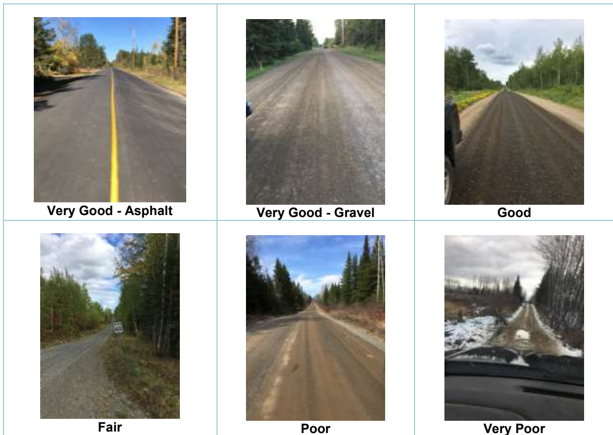
Figure 3.3: Images of Asset Condition - Roads
