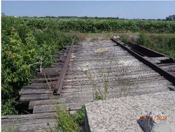
Photograph No. 1: 0718: Driveway over the structure looking east.
