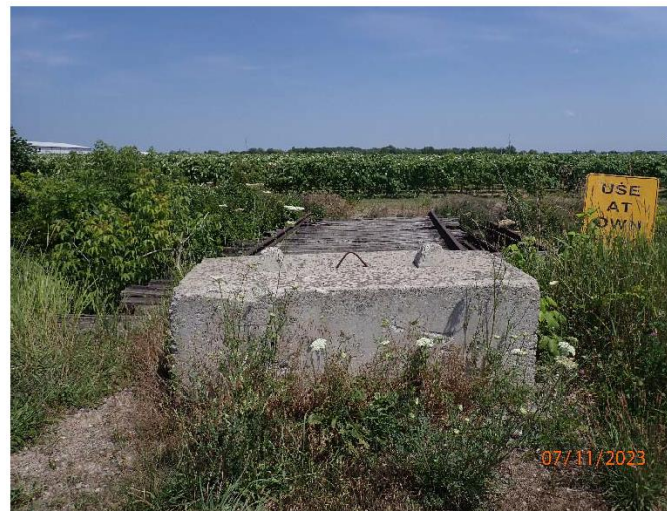
Photograph No. 4: 0722: Concrete barrier at west end.
