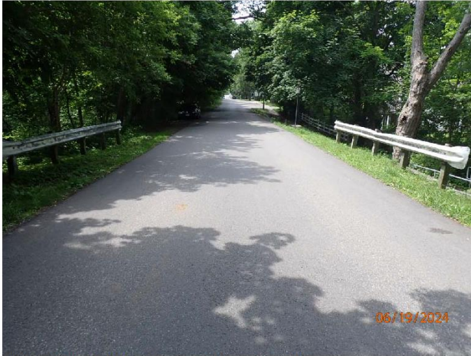
Photograph No. 1: 0419: Roadway over the structure looking south.
