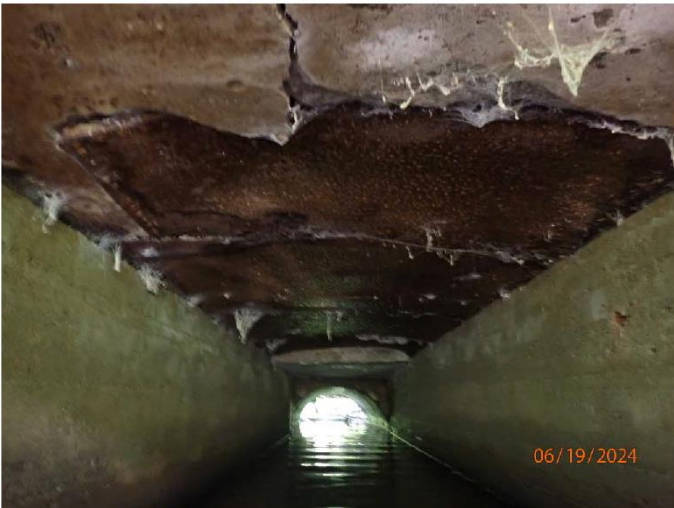
Photograph No. 3: 0442: Interior of west half of structure looking east.
