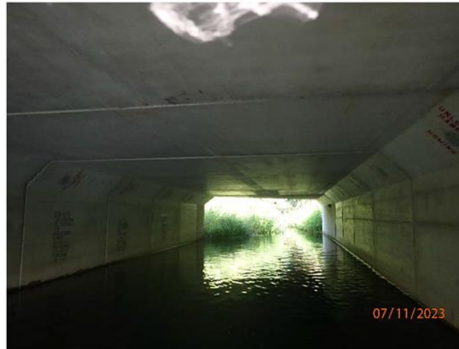
Photograph No. 4: 0258: Underside of the structure looking west.
