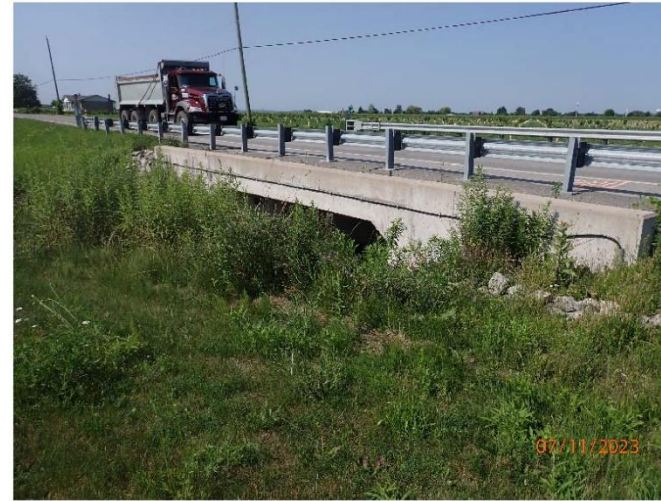
Photograph No. 2: 0248: East elevation.
