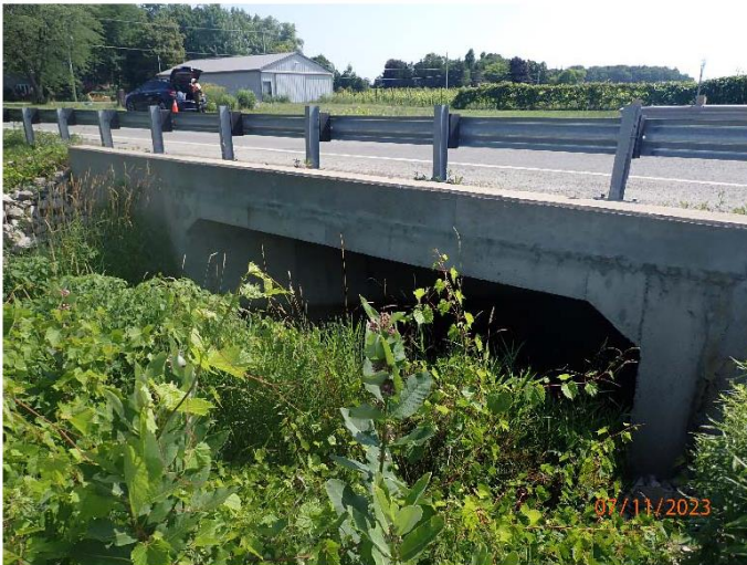
Photograph No. 3: 0285: West elevation.
