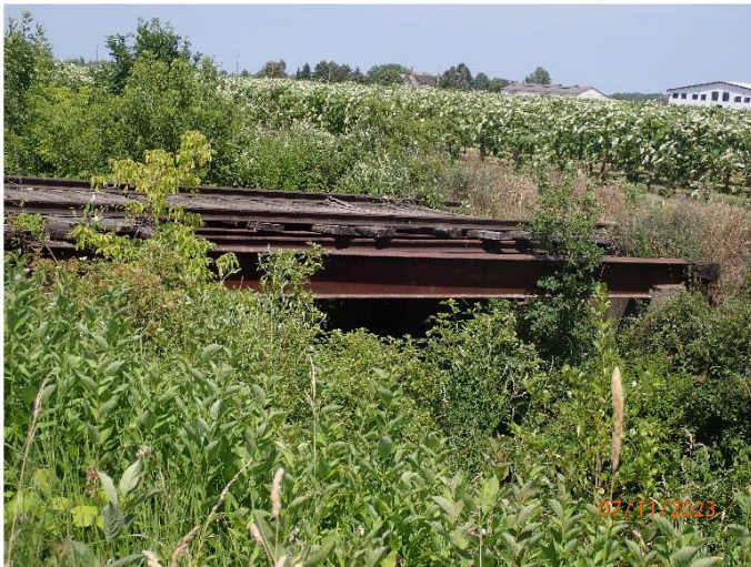
Photograph No. 3: 0725: South elevation.
