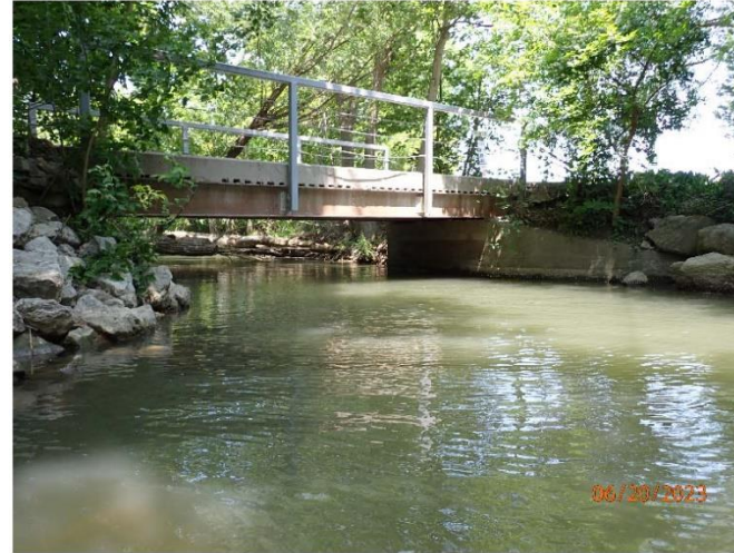
Photograph No. 2: 0771: South elevation.
