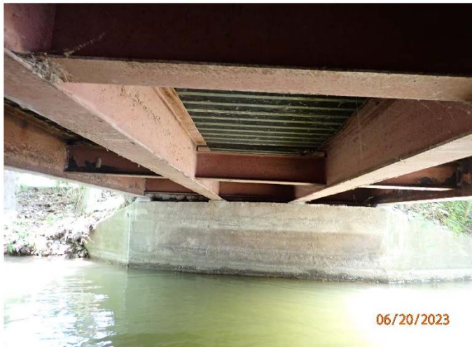
Photograph No. 3: 0788: Underside of the structure and east abutment looking east.
