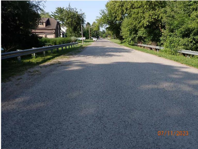
Photograph No. 1: 0012: Roadway over the structure looking south.
