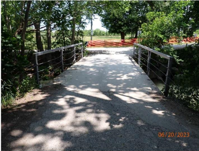
Photograph No. 1: 0766: Roadway over the structure looking east.
