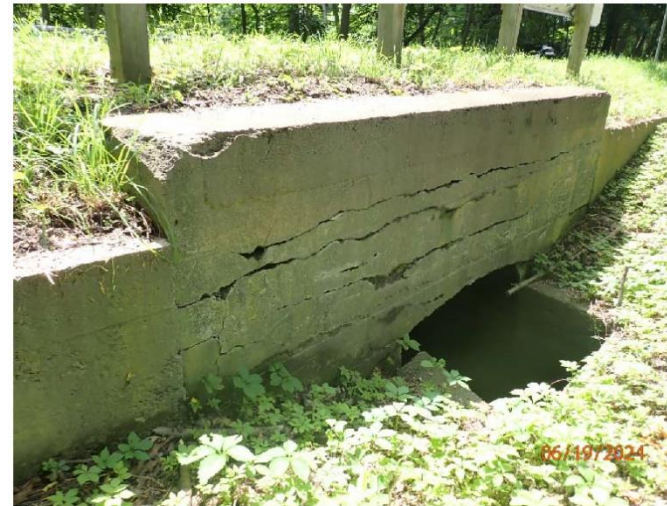
Photograph No. 2: 0437: West elevation.
