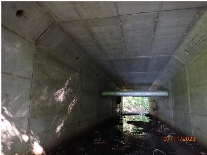
Photograph No. 3: 0050: Underside of the structure looking west.
