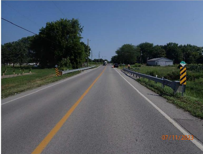
Photograph No. 1: 0227: Roadway over the structure looking north.
