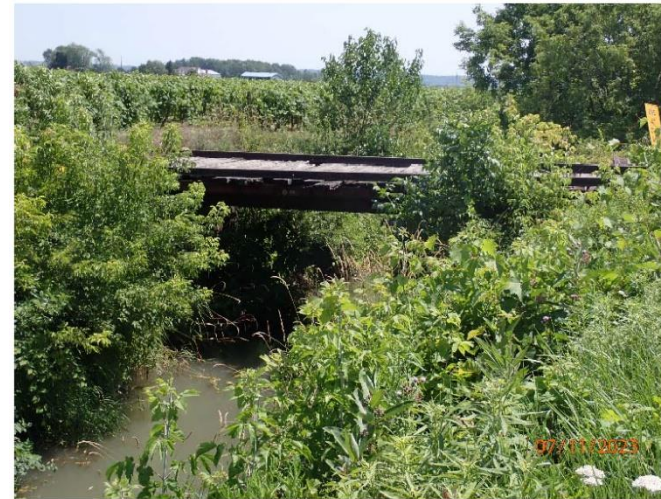
Photograph No. 2: 0724: North elevation.
