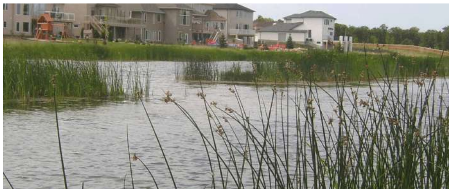
The constructed natural wetlands in Royalwood subdivision (Winnipeg, Manitoba) have replaced standard stormwater retention ponds. Not only are they an environmentally sound solution to water retention, but they also serve as a beautiful focal point and unique recreational and educational resource.
