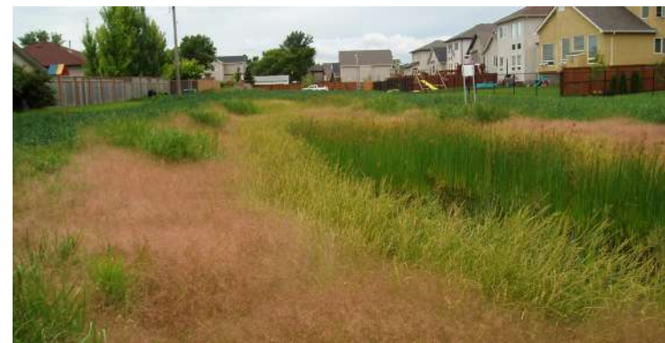
Bio-swale, Seven Oaks subdivision, Winnipeg, Manitoba. Bio-retention systems are designed to mimic processes that occur in the natural environment by filtering and storing runoff water from rainstorms and snow melt, rather than letting it be flushed through the stormwater sewer system.
