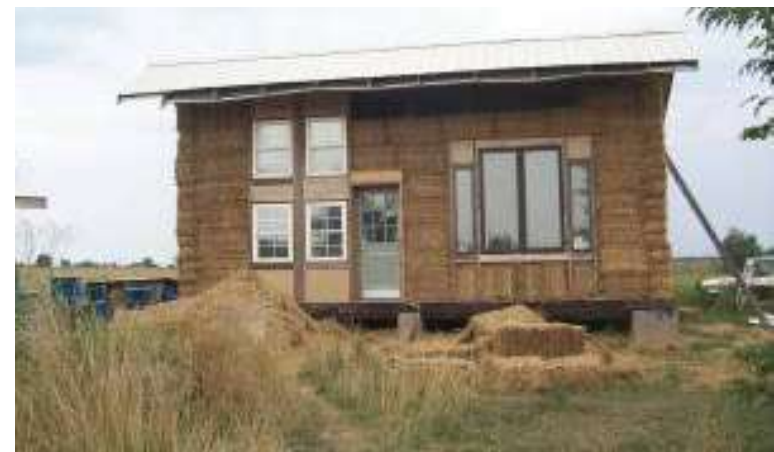
Straw bale construction
