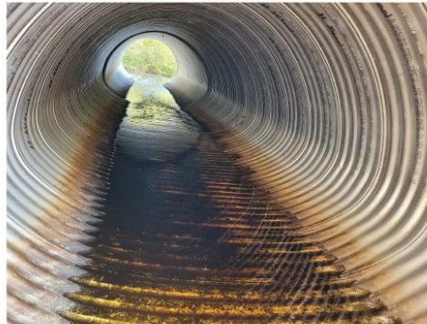
6. Inside South Barrel (looking east)
