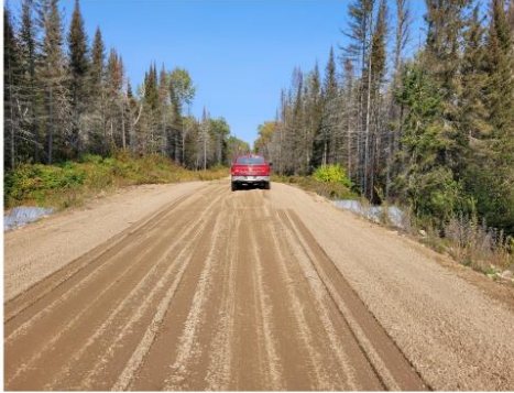
2. South Approach (looking north)
