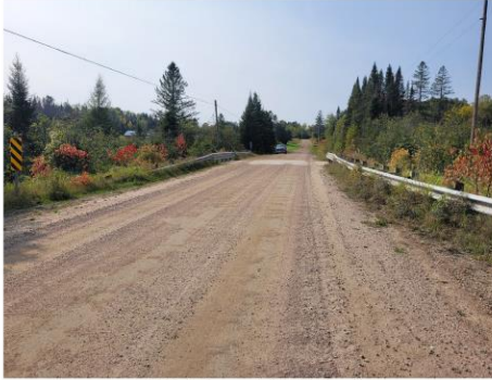
1. East Approach (looking west)
