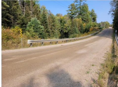
4. North Barrier (looking east)
