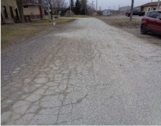
Asphalt (left) and gravel (right) roads in Very Poor condition – no longer functional, general or complete failure
