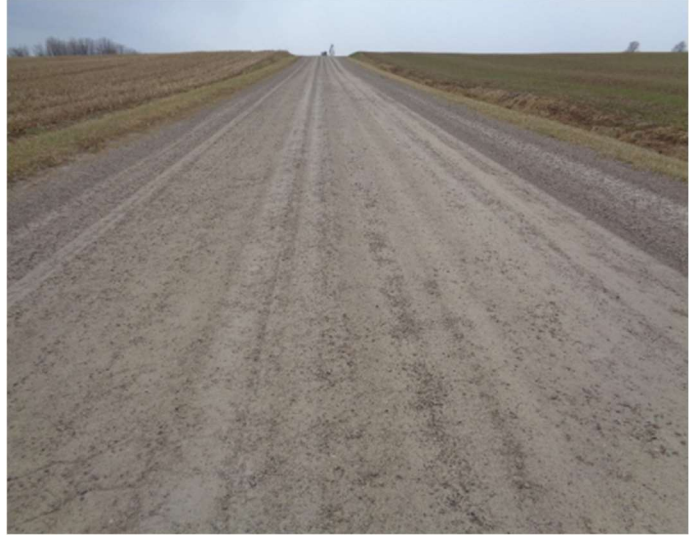
Asphalt (left) and gravel (right) roads in Fair condition – deterioration evident, function is affected
