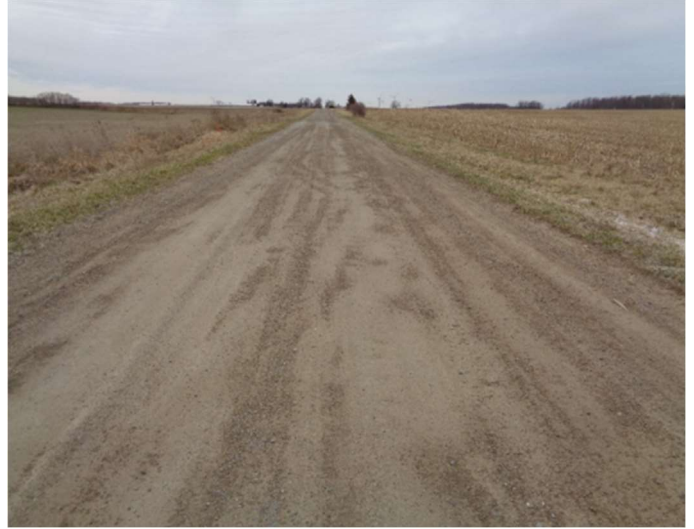
Asphalt (left) and gravel (right) roads in Very Poor condition – no longer functional, general or complete failure
