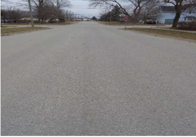
Asphalt (left) and gravel (right) roads in Very Good condition – no noticeable defects
