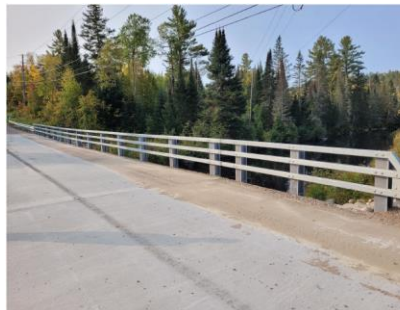
West Barrier Looking South
