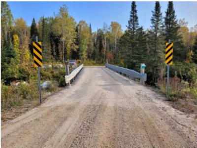
South Approach Looking North
