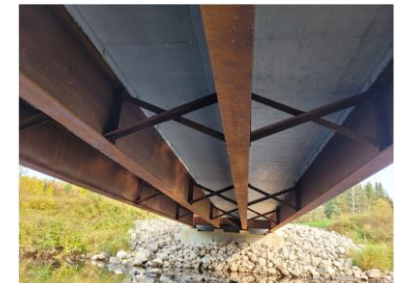
Underside of Bridge Looking North
