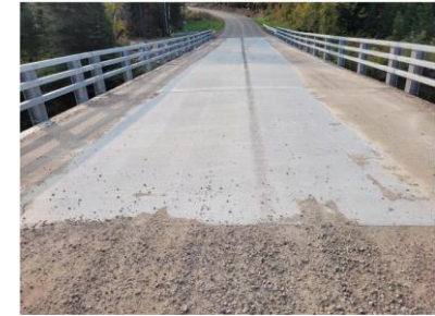
Bridge Deck Looking South
