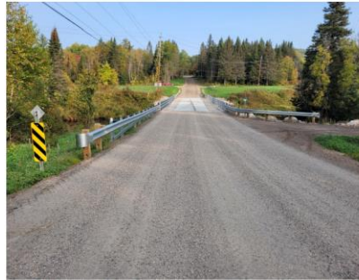
South Approach Looking North
