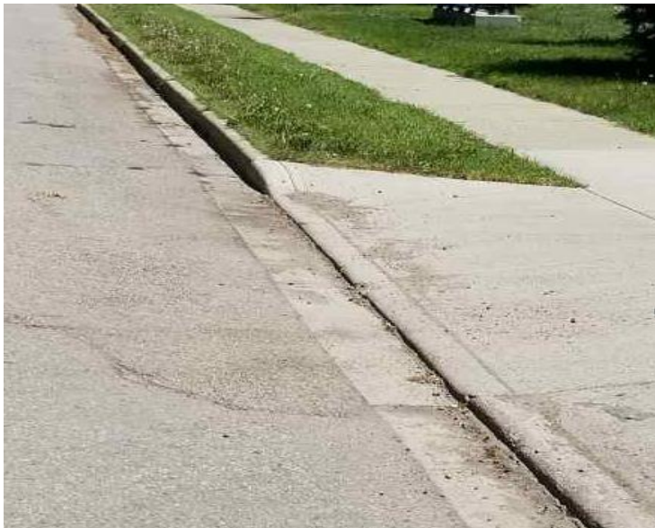
Figure 1 – Curb lowered to allow vehicle access.
