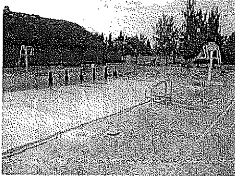
Photo 48: Pool – From The North West
