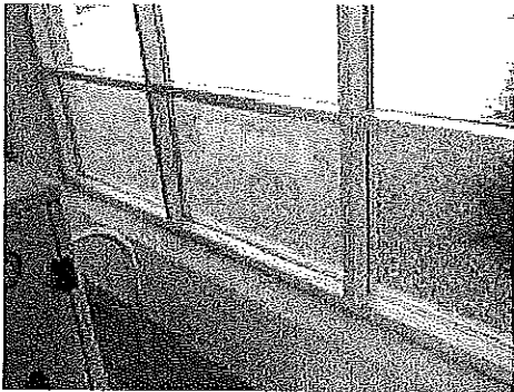
Photo 36: WTP – North Side Windows
