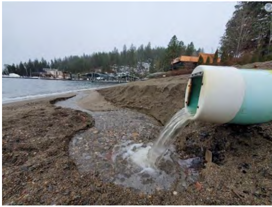
Figure 7. Uncontrolled stormwater outflow causing beach erosion.
