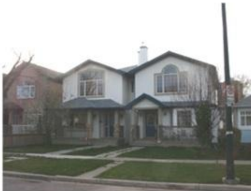
Example of a mirror image semi-detached dwelling with a recessed party wall, creating the illusion that they are two separate dwellings
