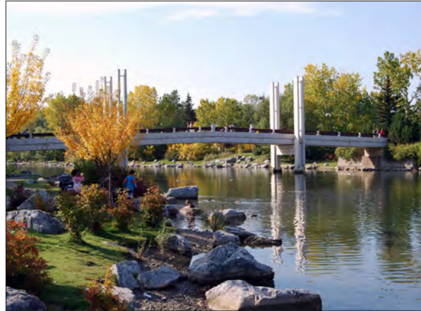
PEDESTRIAN BRIDGE, CALGARY
