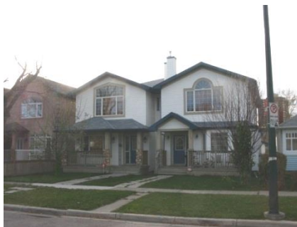
Example of a duplex with a recessed party wall, creating the illusion that they are two separate dwellings.
