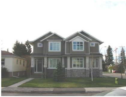
Example of a duplex resembling one large dwelling.
