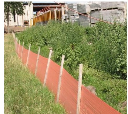
Guideline 2.2.8 Temporary high visibility fencing is required to delineate non-
