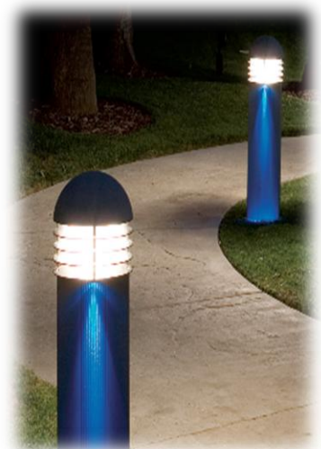
Onsite walkway lighting
