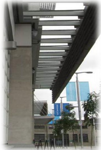
Weather protection for users
