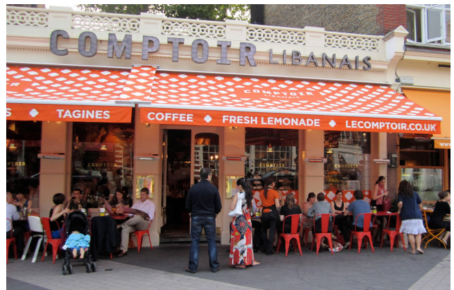
Guideline b, c, and d: Vibrant accent colours help create a welcoming streetscape, with a streetside patio under awnings
