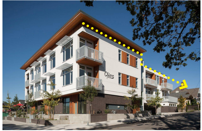
Guideline a and e: Addressing both street frontages and stepping down and back to create a smoother transition to the adjacent, lower density residential area
